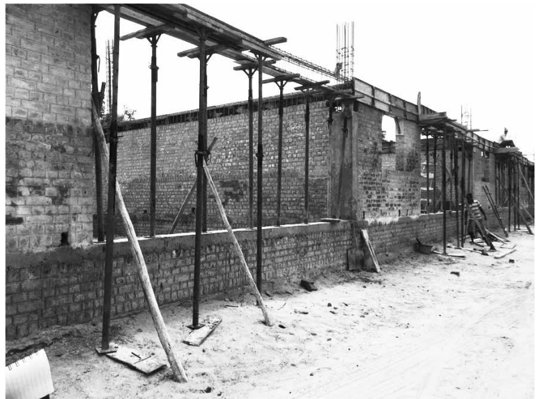
Figure 4.11: Mango pulping unit being constructed by an FPC in Tamil Nadu
